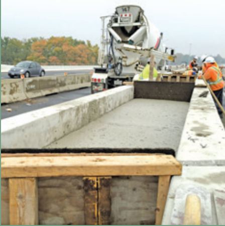
Hwy 7/8 Overpasses (Barrier wall gap filling)
