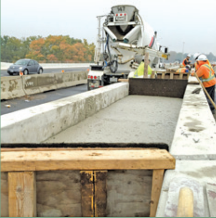
Hwy 7/8 Overpasses (Barrier wall gap filling)
