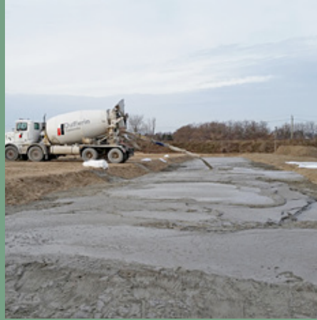
Durham Region Transit Maintenance Facility (Watermain protection and insulation)
