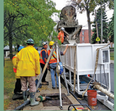
Toronto Gerrard Street Watermain Replacement (Discarded watermain backfilling)
